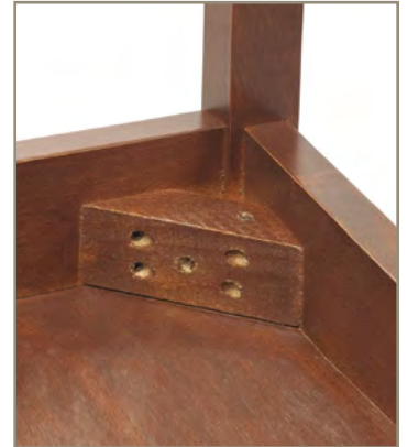
Corner block strengthens corners
